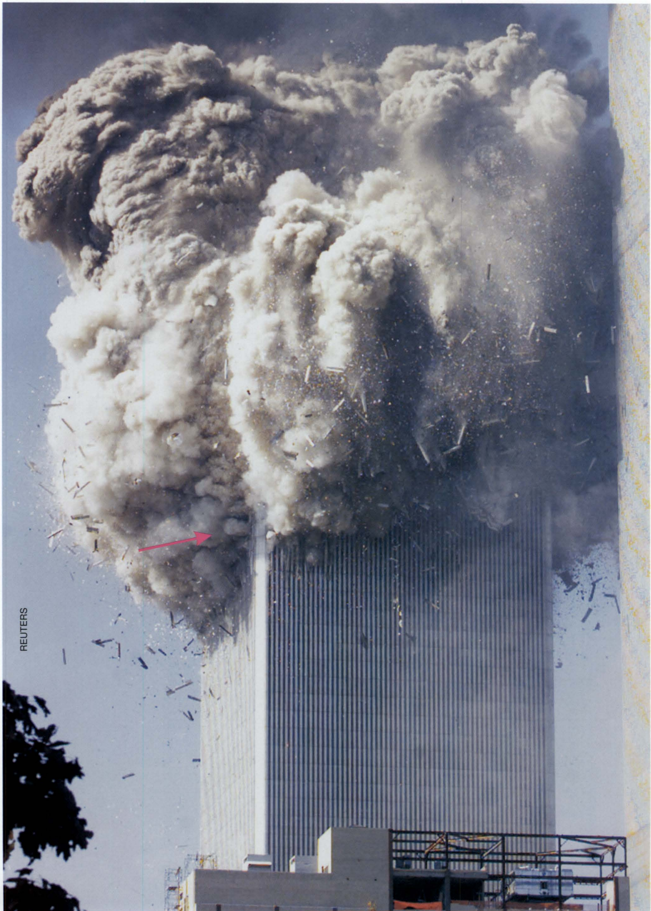
Figure 5-16 The red arrow is pointing to puffs of dust. The significance of the dust will be discussed in Chapter 7
