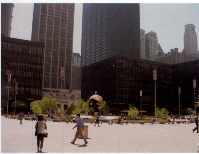
The courtyard. Building 5 is on the left, Building 4 along the right.
