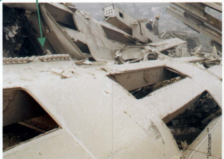
Figure 3-11 The bolts holding the pre-fab units together.
