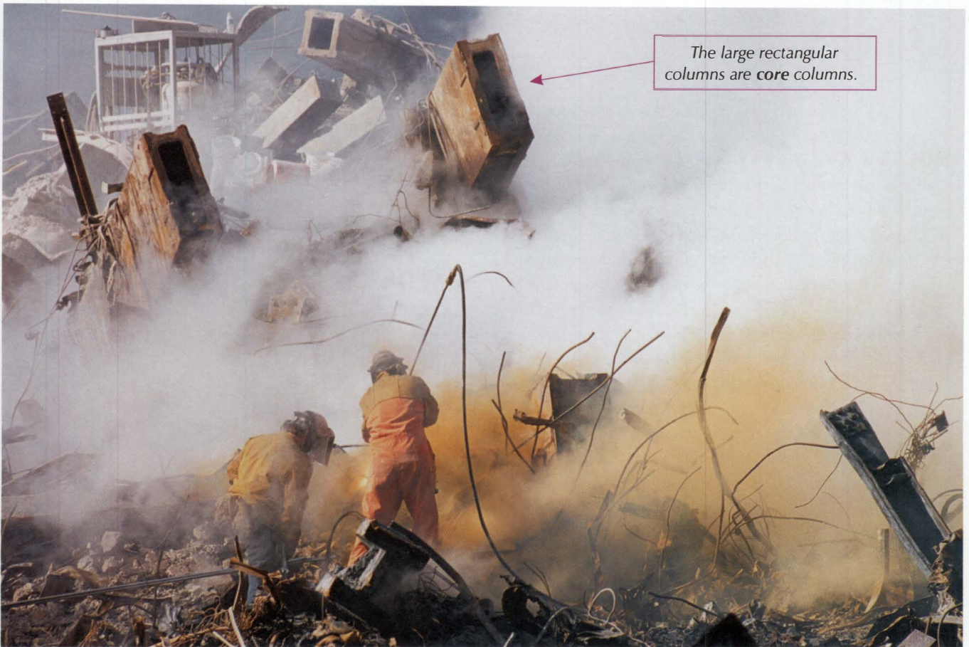
Figure 3-4 The workers are cutting the steel with giant torches.
