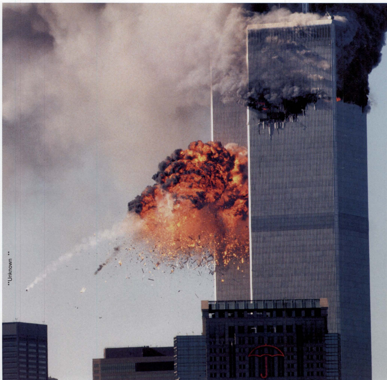
Figure 4-12 This photograph was taken slightly before the one in Figure 4-7. There are only a few flames in the North Tower, and the smoke is very dark. The fires have been burning for only 16 minutes but already most flames have vanished. Why didn't the fire grow over time?
