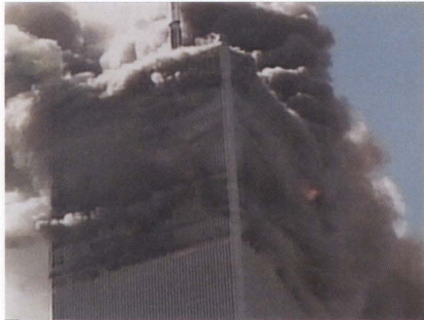
Figure 5-21 The top of the North Tower has dropped a small amount, which means the entire top section has been severed from the base.
