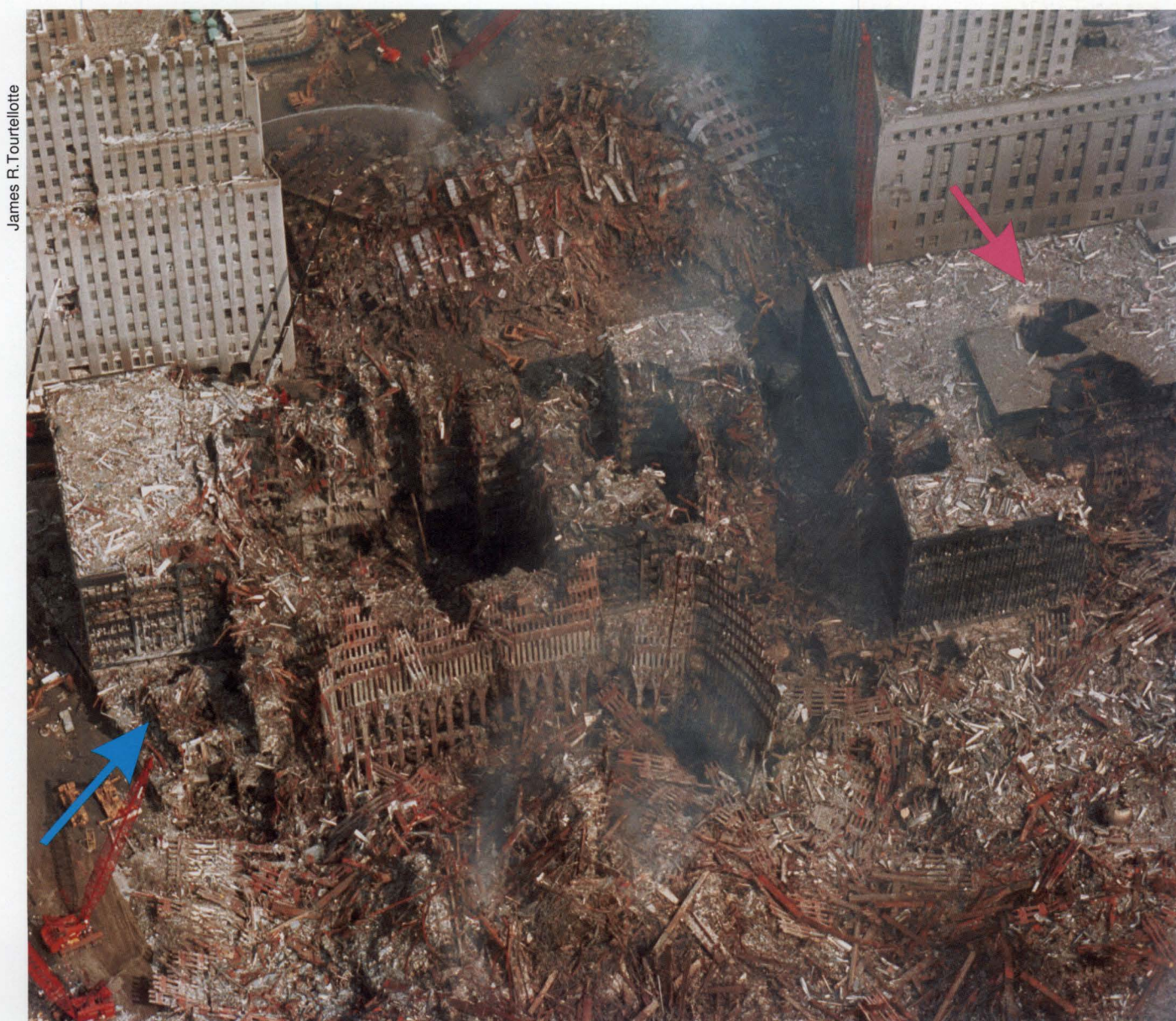
Figure 6-4 The blue arrow shows approximately the angle of the photo in Figure 6-3. Building 7 is the pile behind Building 6. There are two holes in Building 6, and one in Building 5. The red arrow points to a hole in Building 5.
