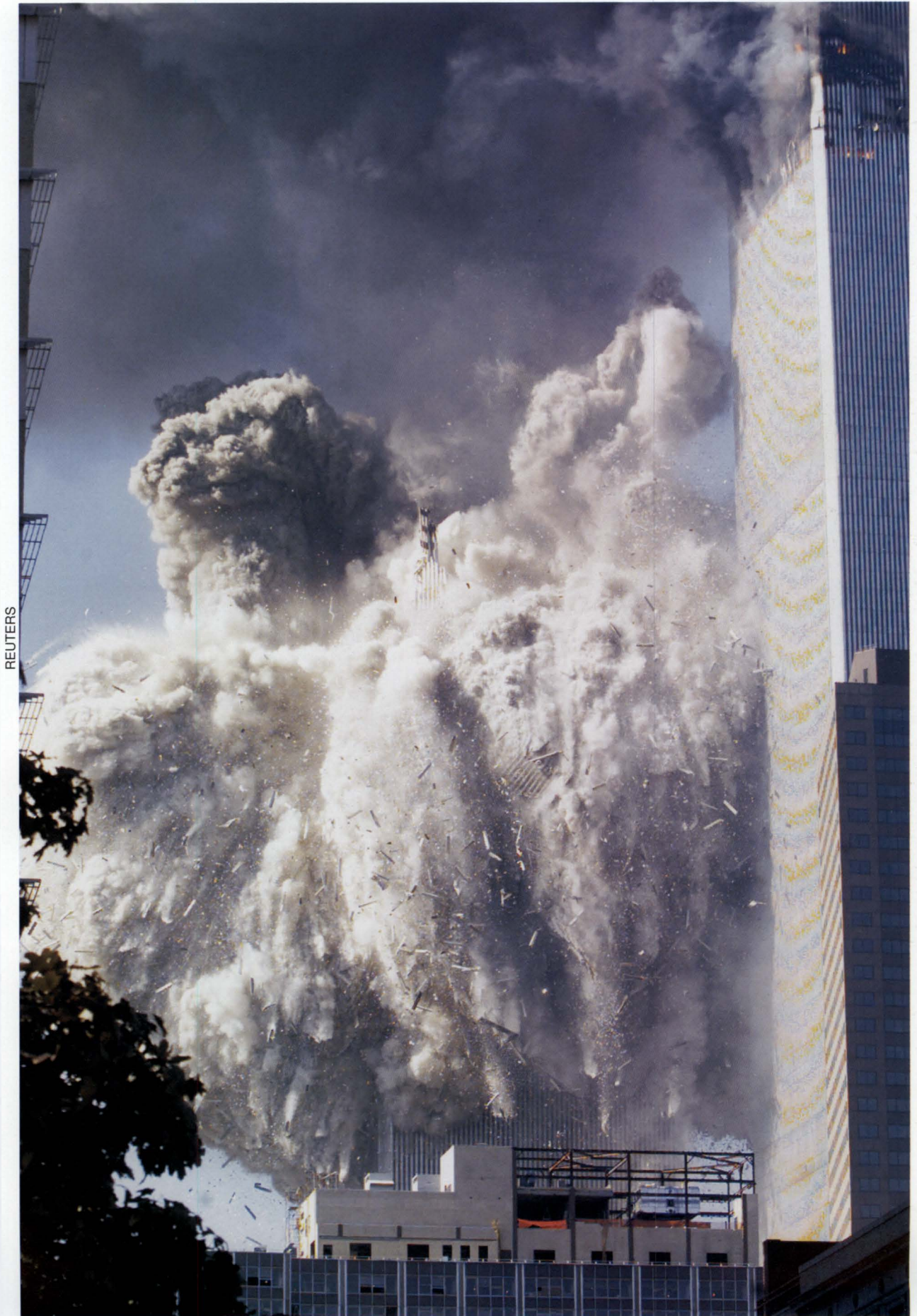
Figure 5-20 The clouds of dust and debris were ejected to perhaps 3 times the width of the tower
